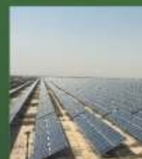
1000MW Quaid-e-Azam Solar Park Bahawalpur Estimated Cost US $1.2 Billion
