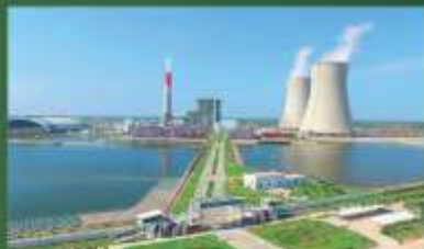
1320MW Sahiwal Coal-fired Power Plant Estimated Cost US $1912 Million
