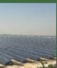
Azam Solar Park Rawalpindi Estimated Cost US $781 Million
