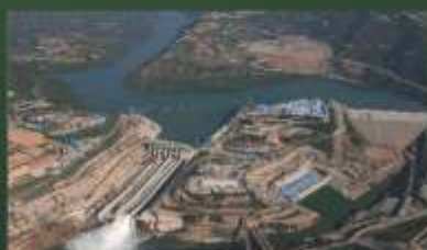
720MW Karot Hydropower Project, AJK/Punjab Estimated Cost US $1698 Million
