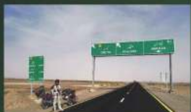
Western Route Hoshab-Awaran Section M8 Estimated Cost PKR 26 Billion
