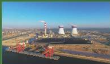
1320MW Coal-fired Power Plant at Port Qasim Karachi Estimated Cost US $1912 Million
